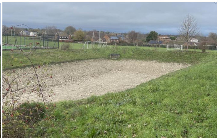
Attenuation basin at Dauntsey's School
