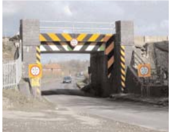
The railway bridge at Littleton Panell
