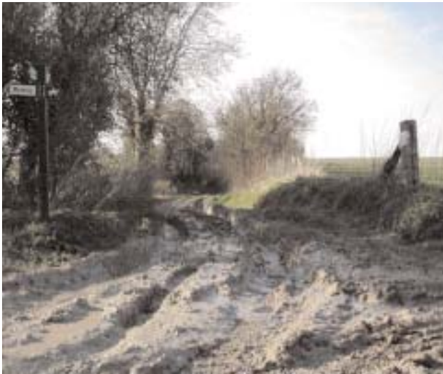
Bridleway near The Warren damaged by 4 x 4 vehicles
