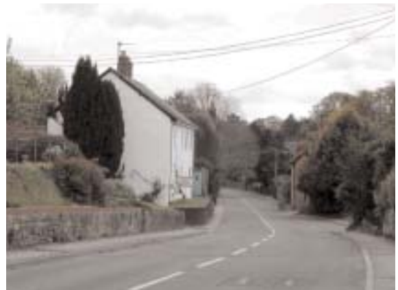
High Street Littleton Panell
